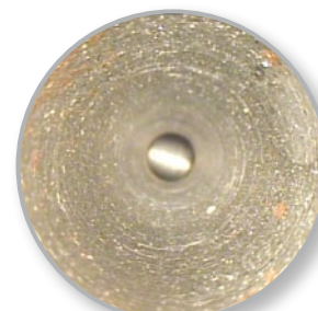
Deposits in pipe
